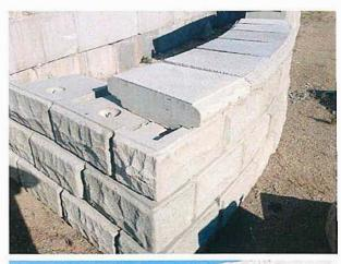
Recessed Blocks available in all shapes. Use to put topsoil up to face of block. No cap needed
